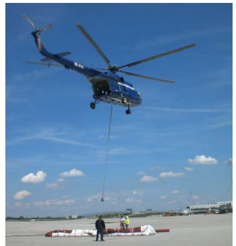
In part, the membrane fields having a package length of 25 m had to be transported onto the roof by means of helicopter.
