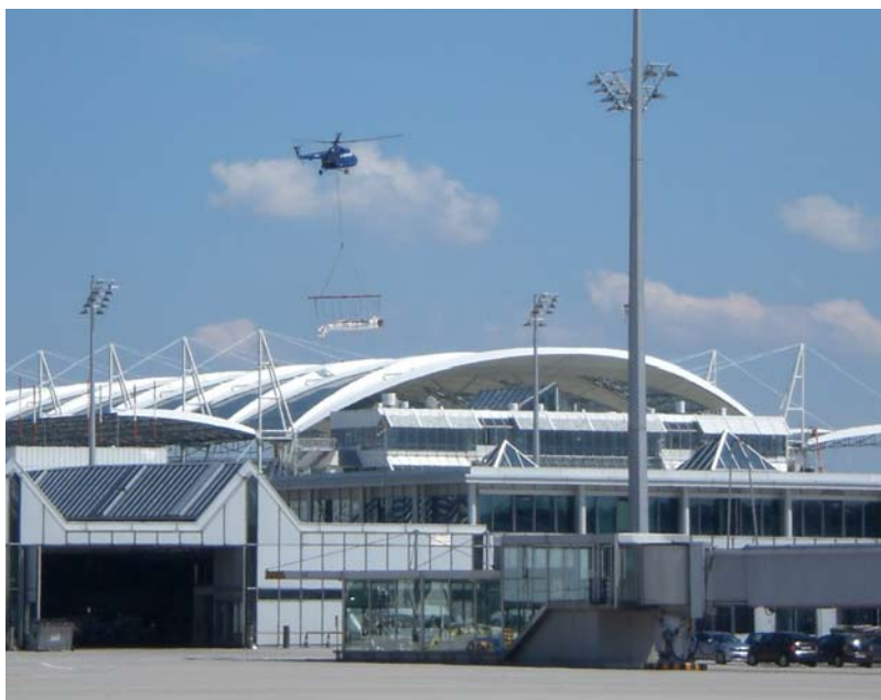
In part, the membrane fields having a package length of 25 m had to be transported onto the roof by means of helicopter.
