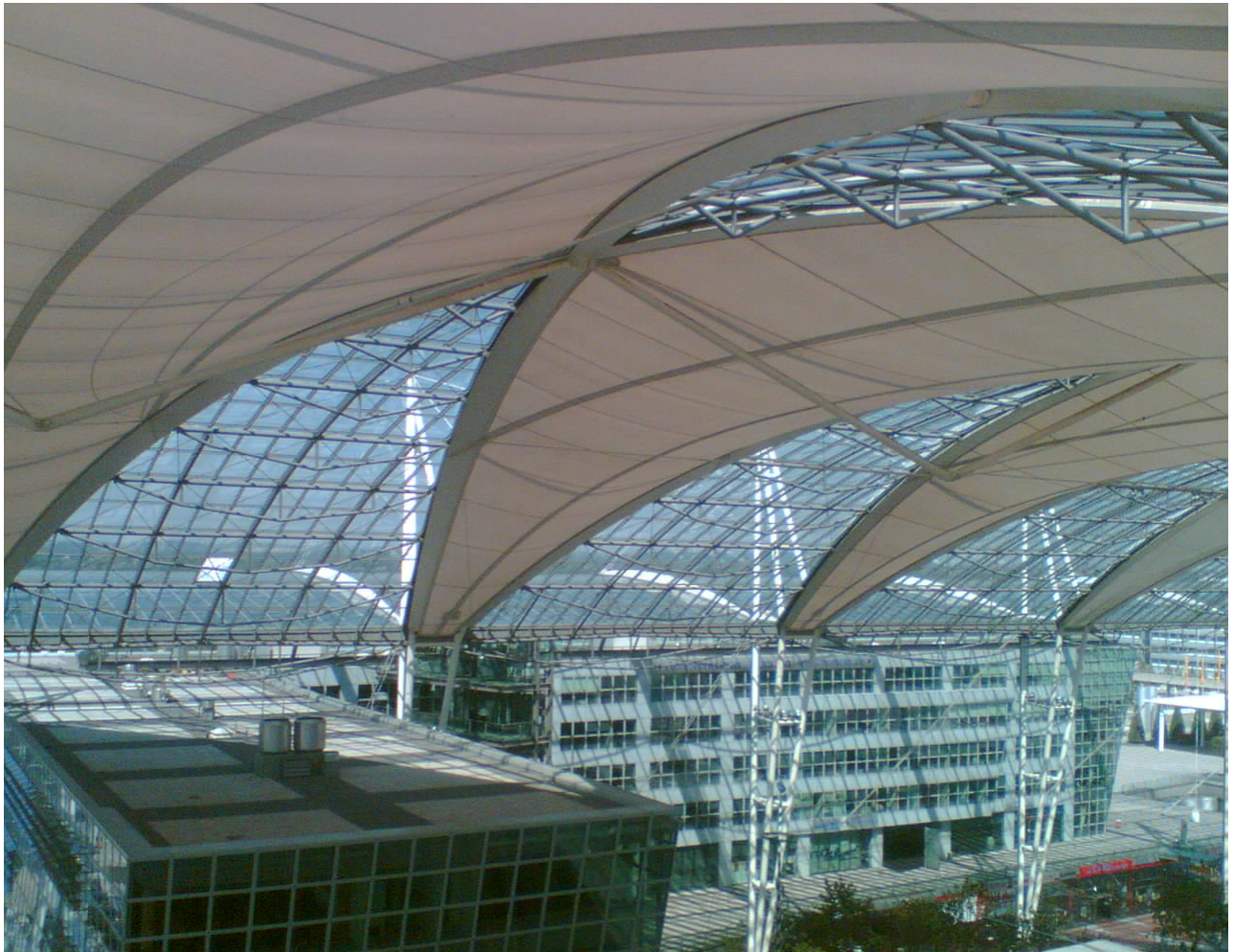
In part, the membrane fields having a package length of 25 m had to be transported onto the roof by means of helicopter.
